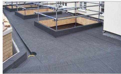
**Fig. 3. Moisture proofing using asphalt**
