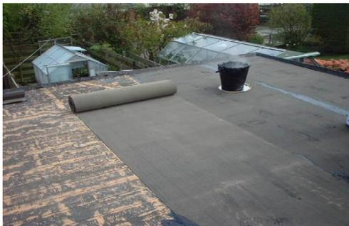
**Fig. 2. Moisture proofing using bitumen**
