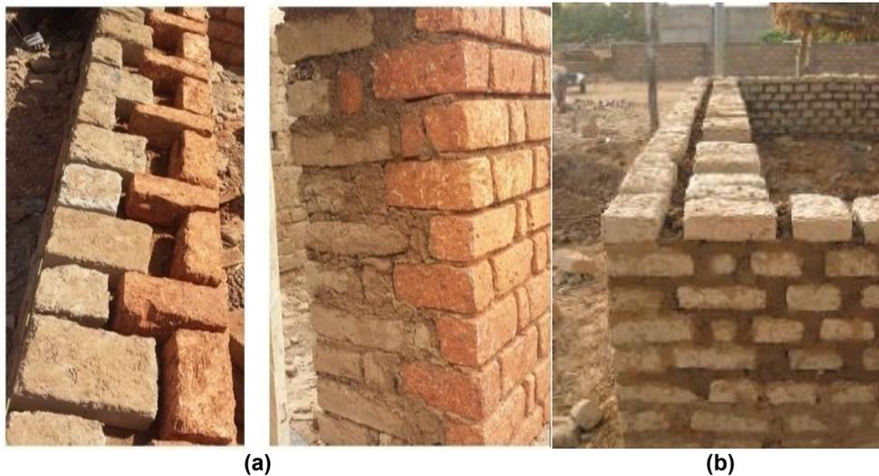
**Fig. 4. (a) Image illustrating the mixed structure of the walls on the East and South sides; (b) Image illustrating a wall bearing a Nubian vault made of adobe [9]**
